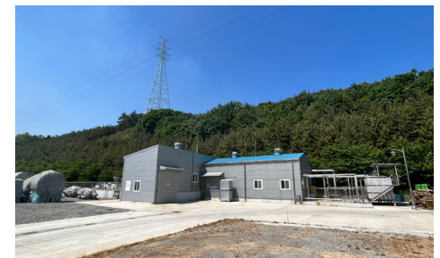
Daesan Plant Wastewater Treatment Facility
