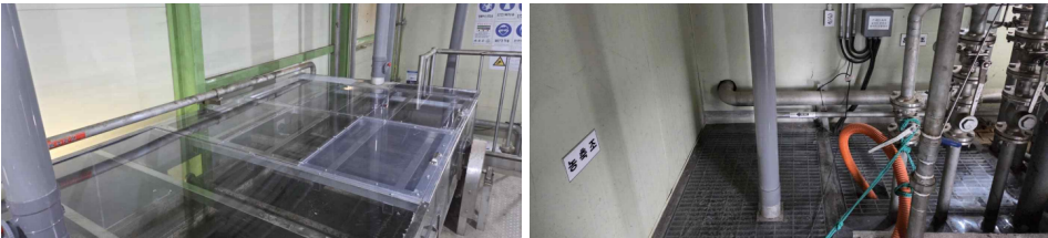
Installation of Hazardous Gas Capture Facilities at the Wastewater Treatment Plant
