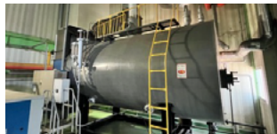
Low-NOx Boiler (10 tons)
