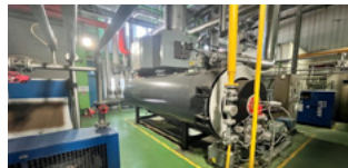
Low-NOx Boiler (3 tons)
